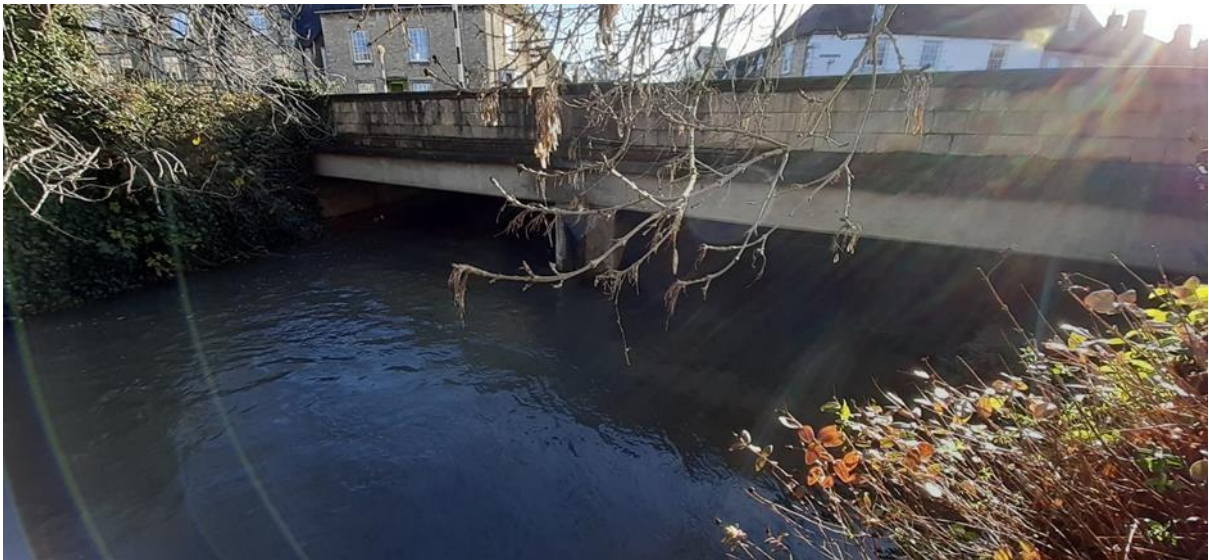
Upstream of Bridge
