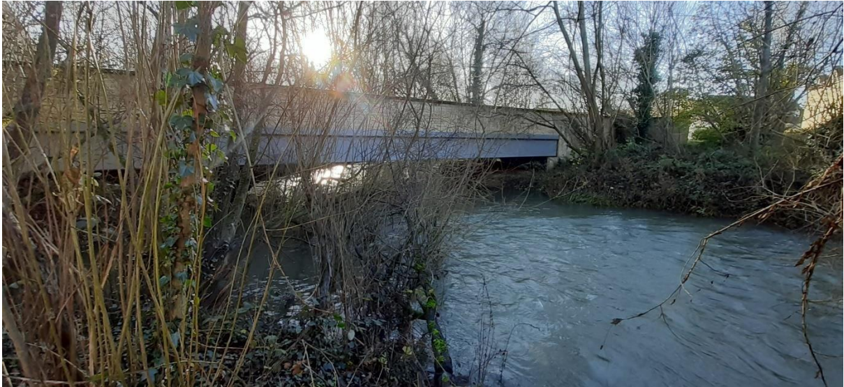
Bridge at New Bridge Street, Aquarius Site access
